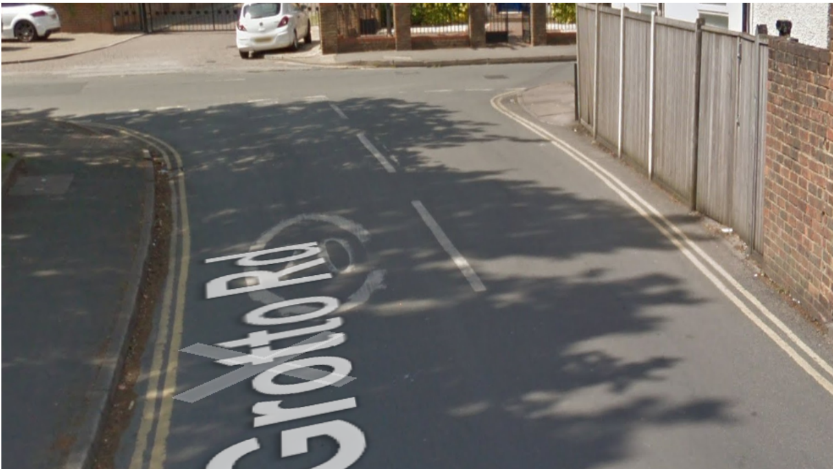
Fig 3. Section of Grotto Road with no footway viewed from Grotto Road
